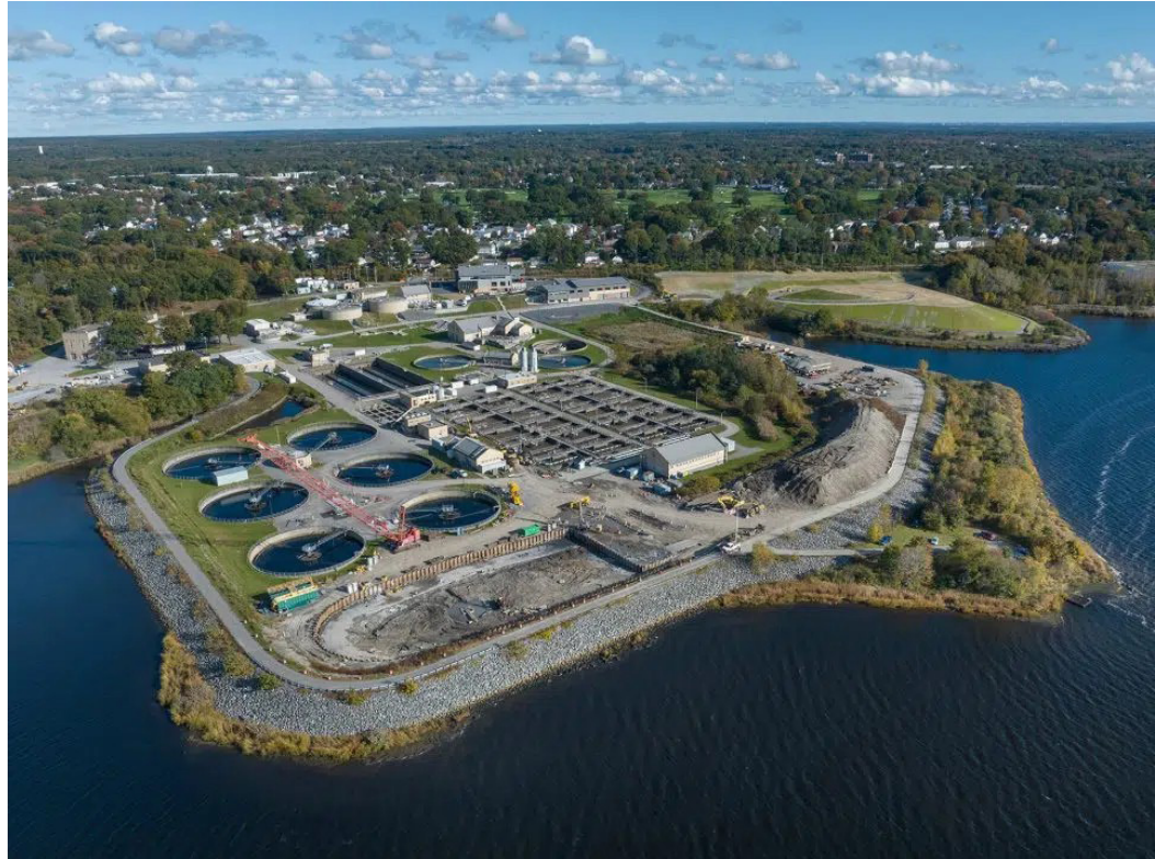
Narragansett Bay Commission's Bucklin Point Wastewater Treatment Facility, where Central Falls' wastewater and stormwater is treated. Image: DOC
