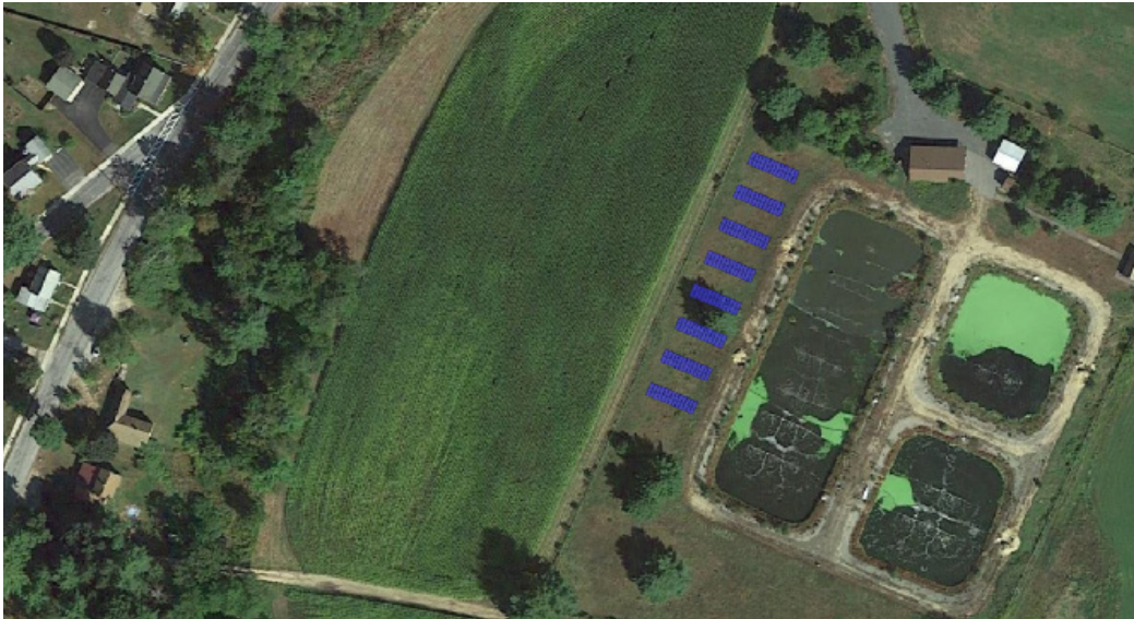
Rendering of the Solar Array at the Swanzeay Wastewater Treatment Facility. Image: Revision Energy
