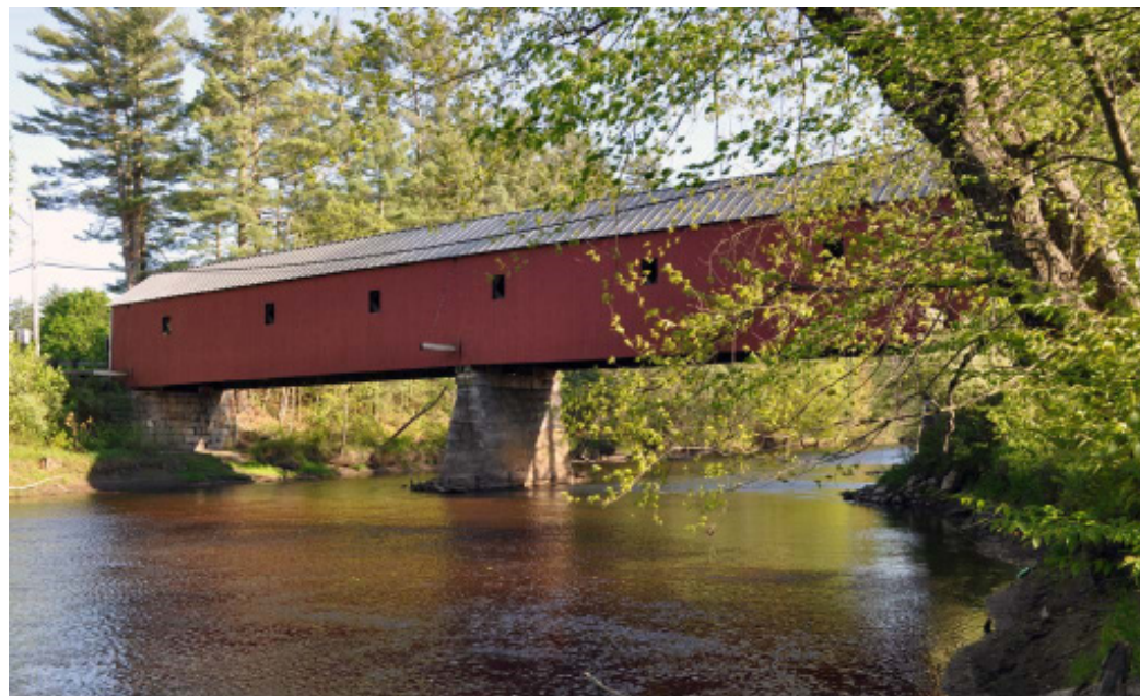
Cresson Covered Bridge, Swanzey, NH. Image: the Greater Monadnock Collaborative
